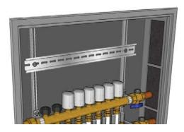
Install a DIN rail on-surface or in the heating circuit distributor cabinet or use an existing one.
